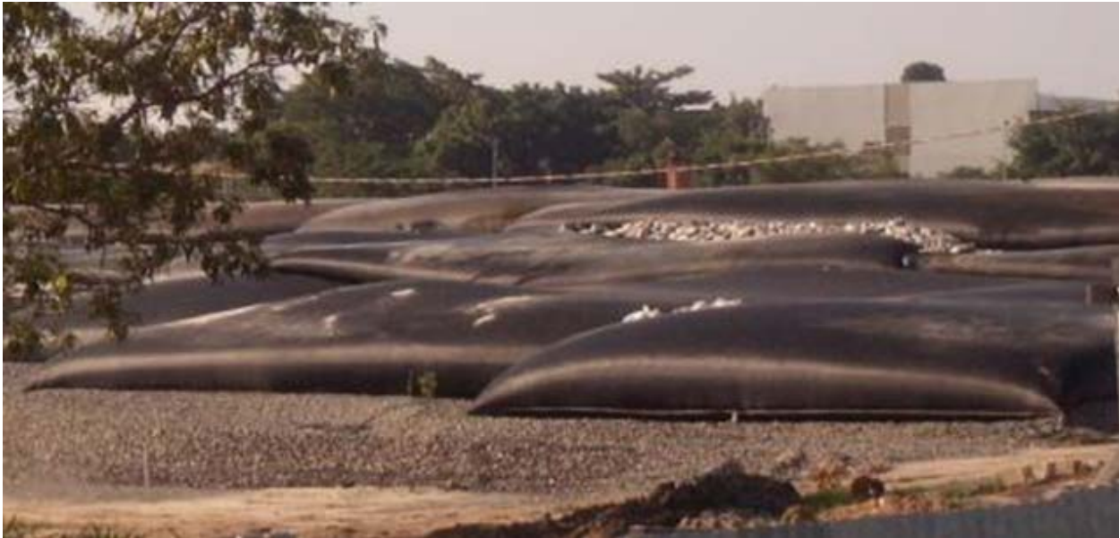
Figure 18-5: Synthetic pods that could be used for tailings disposal. In the case of Berlin, such pod-fields would be covered with a layer of soil thick enough to mask any radiation that may emanate from the tailings
